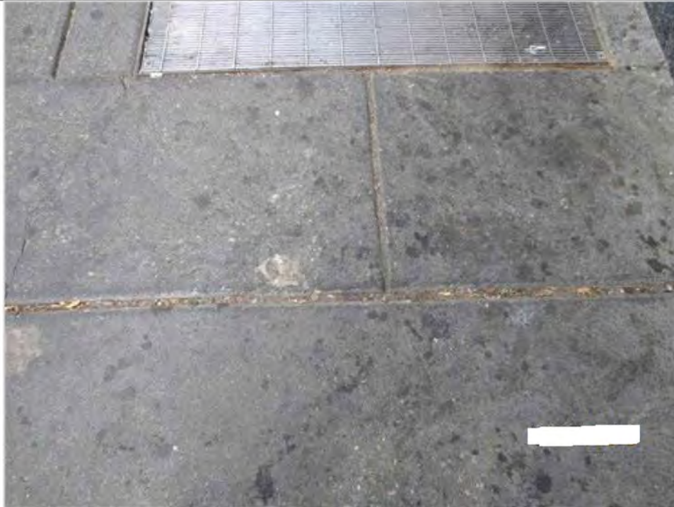
Expansion Joint in Sidewalk
