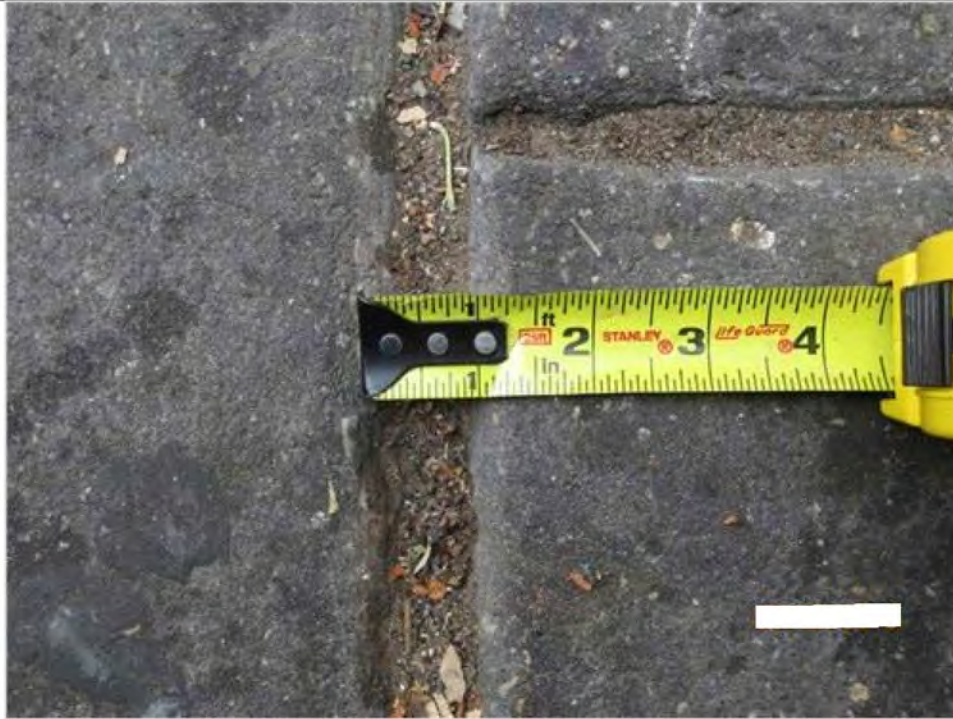
Sidewalk Expansion Joint
