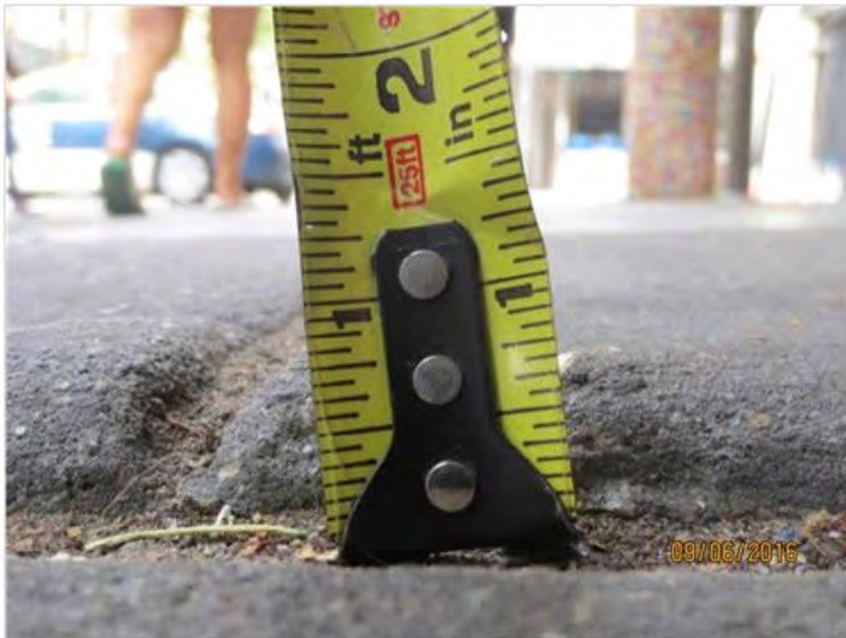
Height of Sidewalk Expansion Joint / North to South
