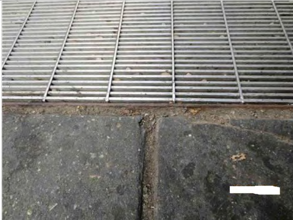
Sidewalk Grate / North to South
