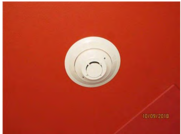
Typical Heat Detector
