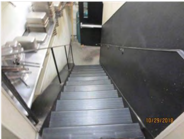
Stairway to Basement Level
