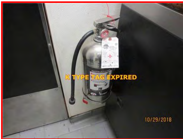
K Type Extinguisher / EXPIRED Tag
